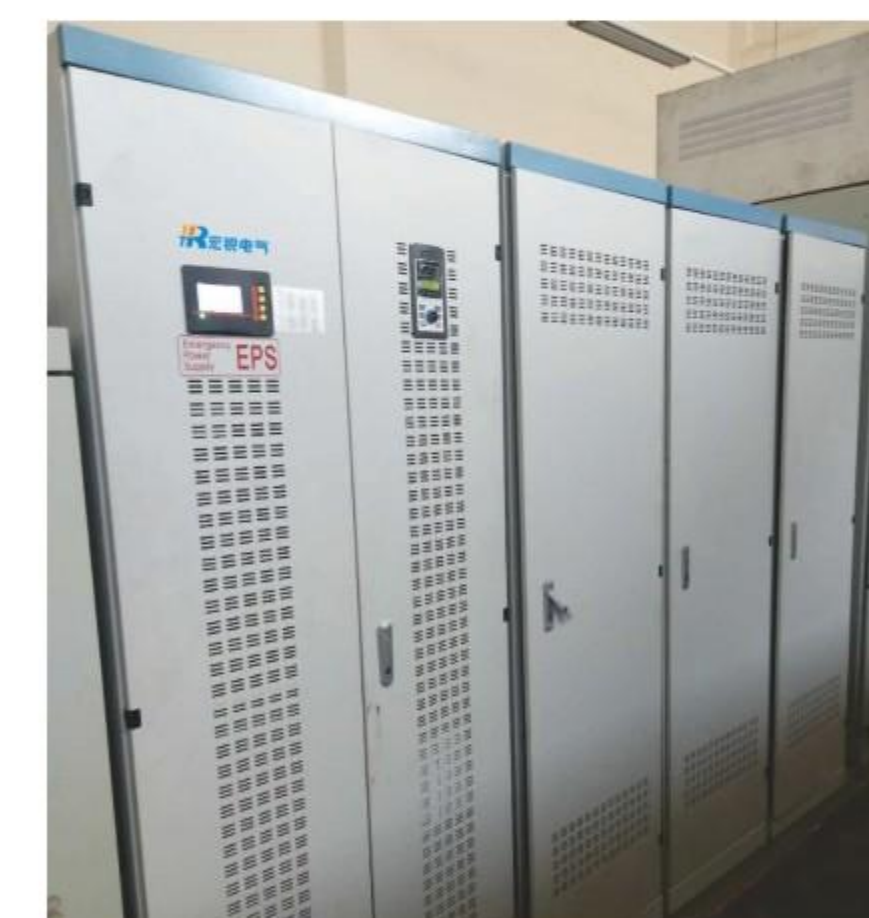
• The electrolysis workshop project of United Copper Industry
